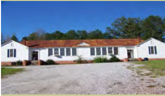
Woodworking Education Center 10544 Hwy 17, Maylene, AL 35114
